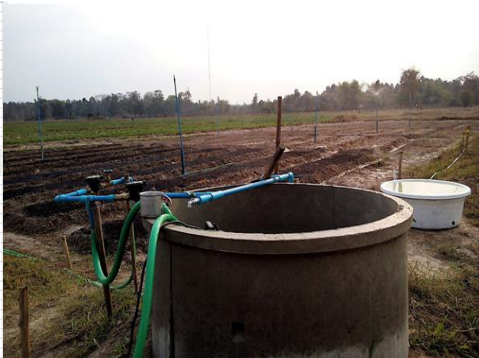
Figure 10: Testing the Irrigation System Prior to Planting Seeds
